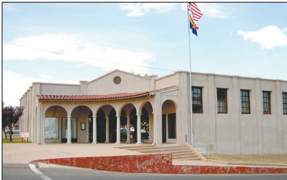
Clarkdale Town Hall
