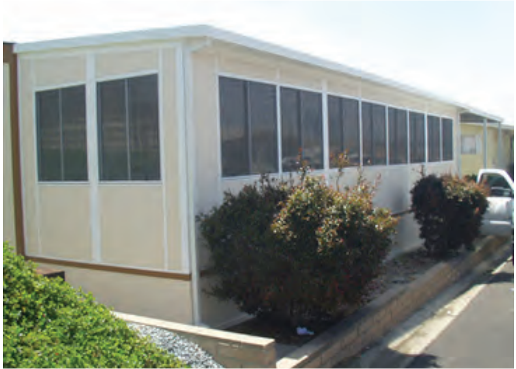
It is important to re-level a mobile home about every other year to keep it in top shape structurally, like the home shown here. (Courtesy/Jordan Mobile Home Service)
